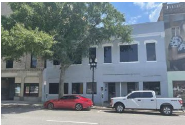
Figure 1. 120 E. Forsyth St (Current Condition)
