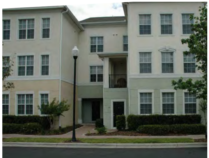
Do Not - Ground level units are missing the additional privacy created by raised footprint.
